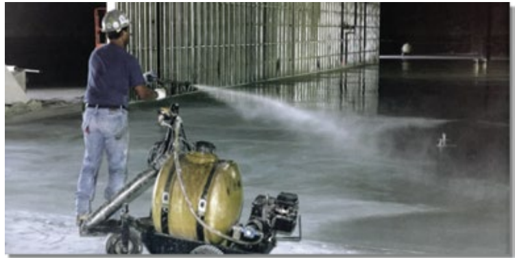
Concrete Cure & Seal WB20 can be sprayed, rolled or applied by brush.
