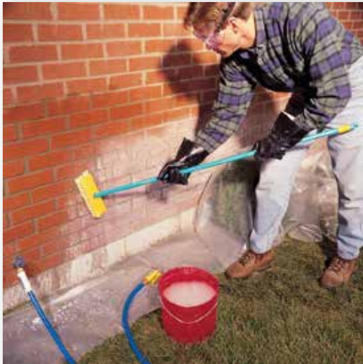
Renew aged brick - Cleans efflorescence and mineral deposits
